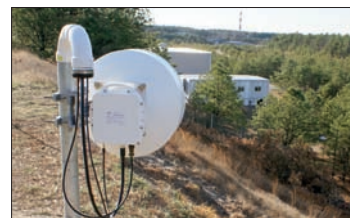
Fig. 3. Schematic of stochastic cooling in RHIC (above). Longitudinal signals are sent via microwave links (right) and transverse signals by fibreoptics in the tunnel. (Image credit: BNL.)
